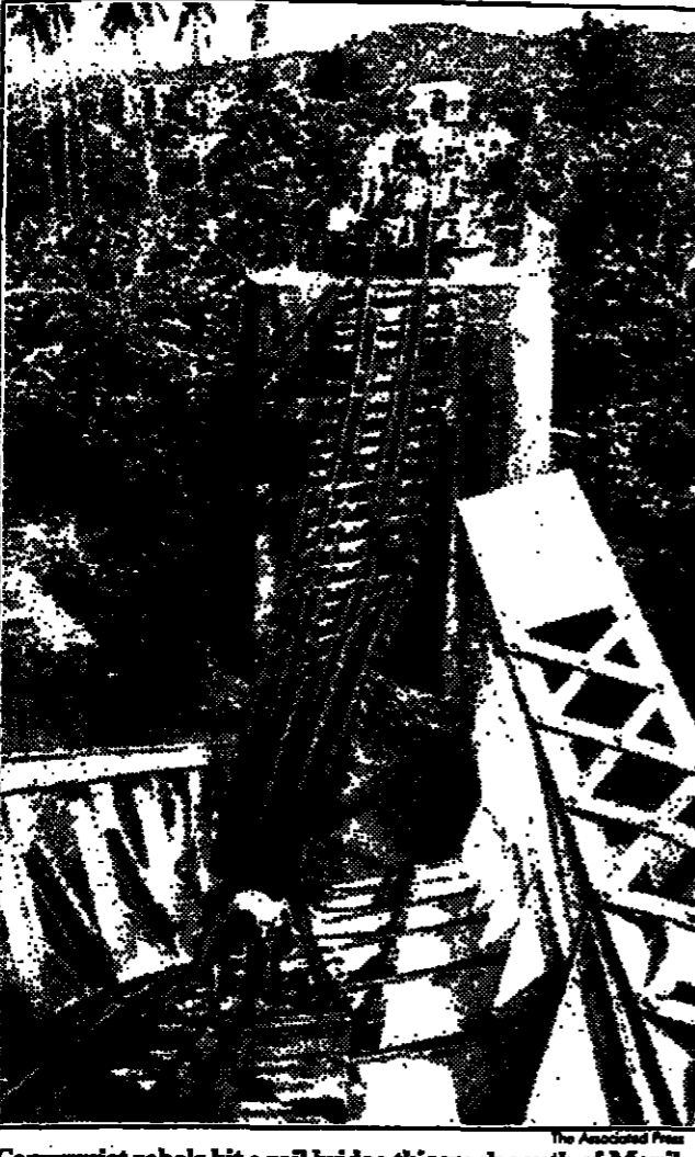
Communist rebels hit a rail bridge this week south of Manila.
